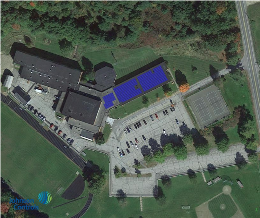
Middle/High School: 168kWdc
